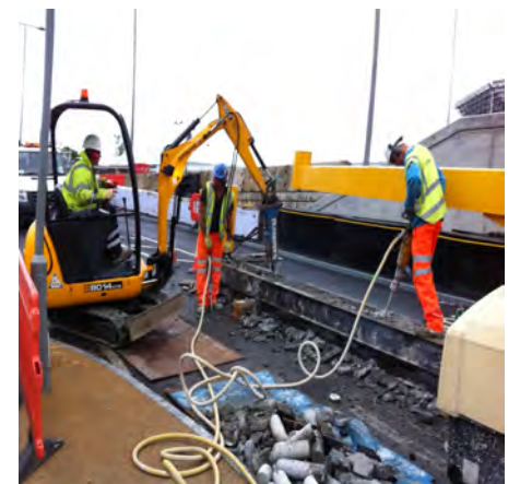
Cleaning off concrete ready for re-use
