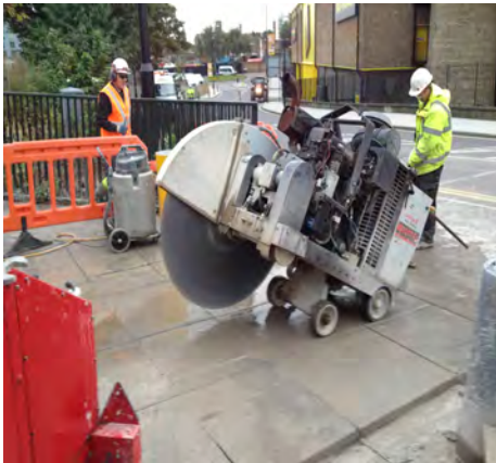
Concrete cutting - 1.2m diameter floor saw
