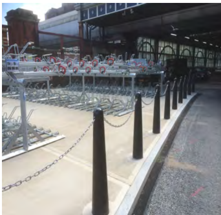
Waterloo - Completed Works
