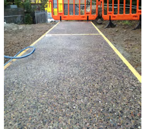
Test panel - Exposed aggregate finish
