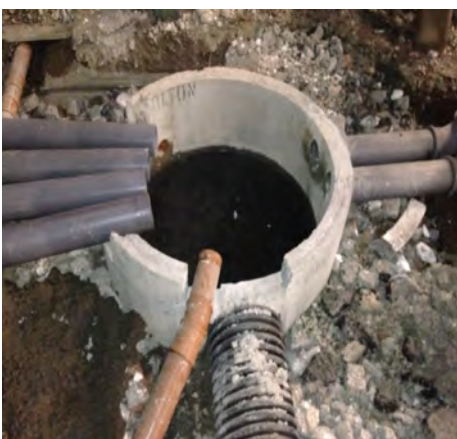
Termination into 1200mm Manhole
