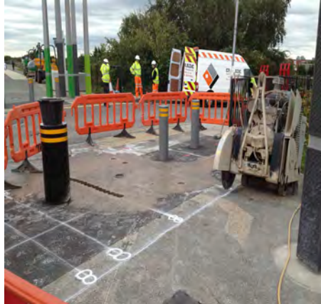
Stitch Coring concrete over shallow utilities
