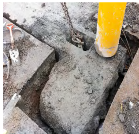
Extracting the gate (12t)
