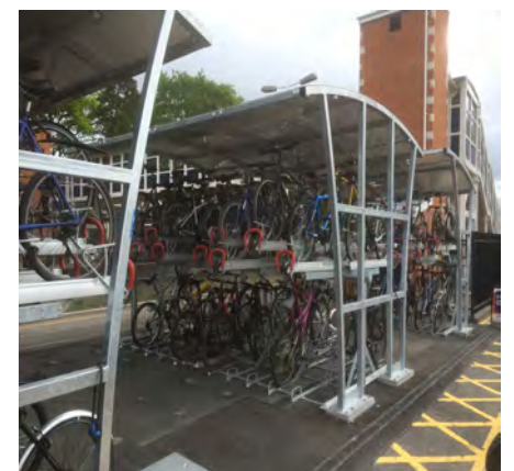
Farnborough Station - Completed works
