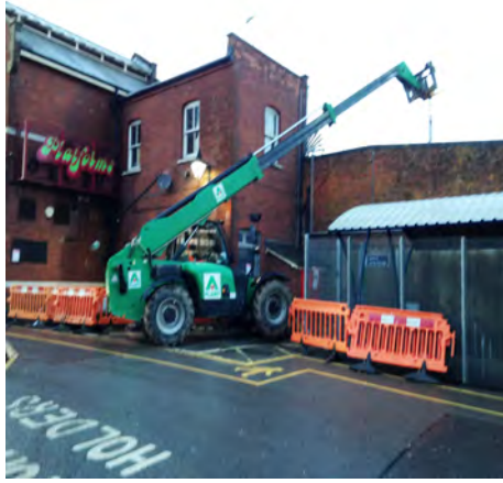
Basingstoke Station - Only access to platform using telehandler
