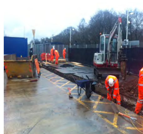
Excavating for ducts and RC bases
