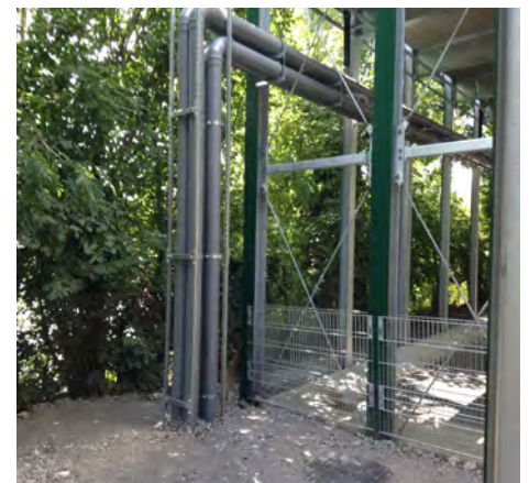
Uni-Strut Structure in place
