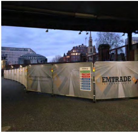
Waterloo Station- Site set up
