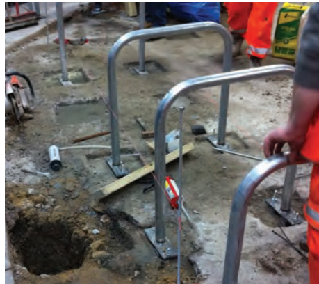
Salisbury Station - Cellar exposed
