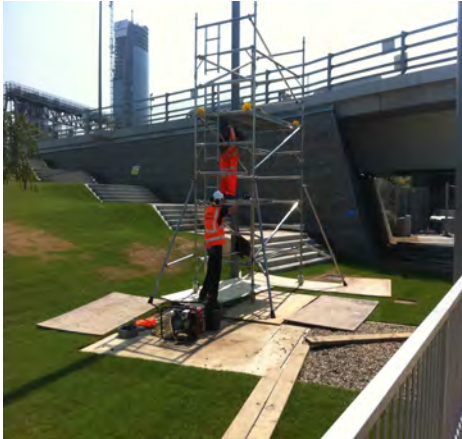
Installing PA System
