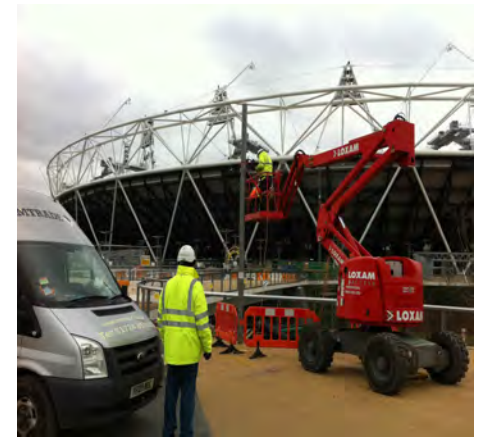
Installing PA System
