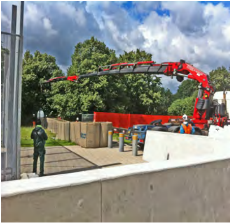
150 ton truck crane working at 35m
