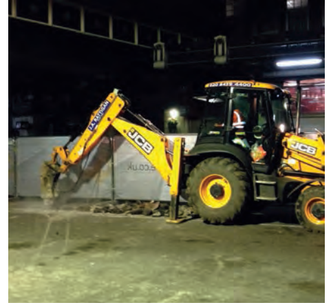
Night Shift Excavation For New Kerb Line
