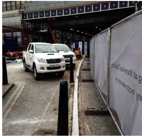
Waterloo Station- New kerb line
