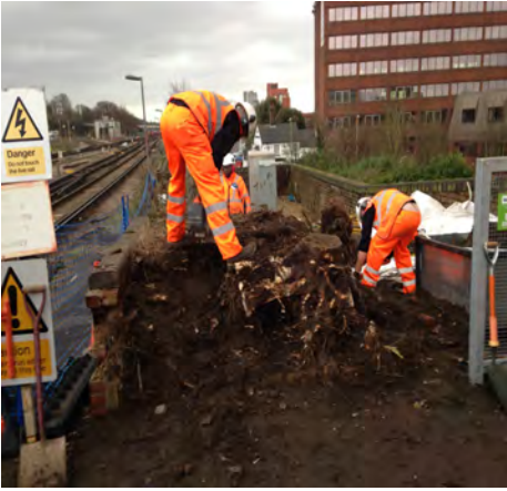
Basingstoke Station - Manual removal of tree roots (Engineering hours)
