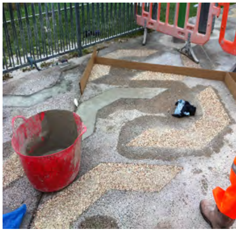
Re-instating concrete artwork
