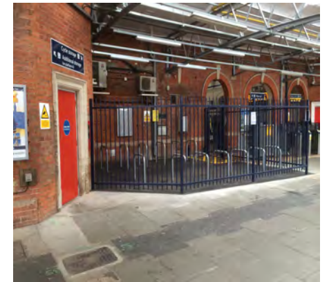
Salisbury Station - Completed Works
