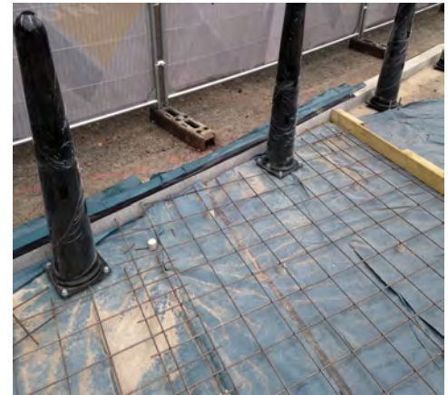
Bollards modified and surface mounted
